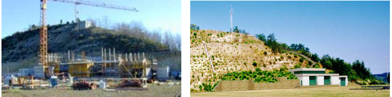
Figure 15 – Work in progress and future result
